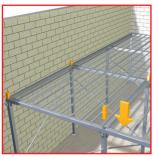
To raise the load deck remove any handrails and from the base, insert connection spigots into all four corners of one complete deck section
